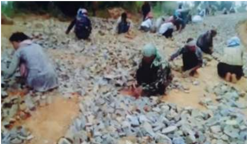
b) Soiling and metalling in Chungtia village under Ongpangkong South RD Block of Mokokchung district.
