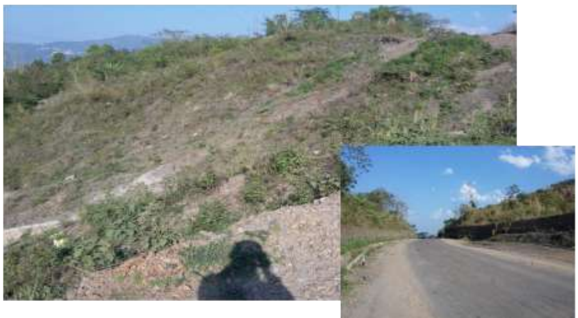
Plates 5.4.1 Landslide at NH 39 and retaining wall constructed on both side of the road to control landslide
