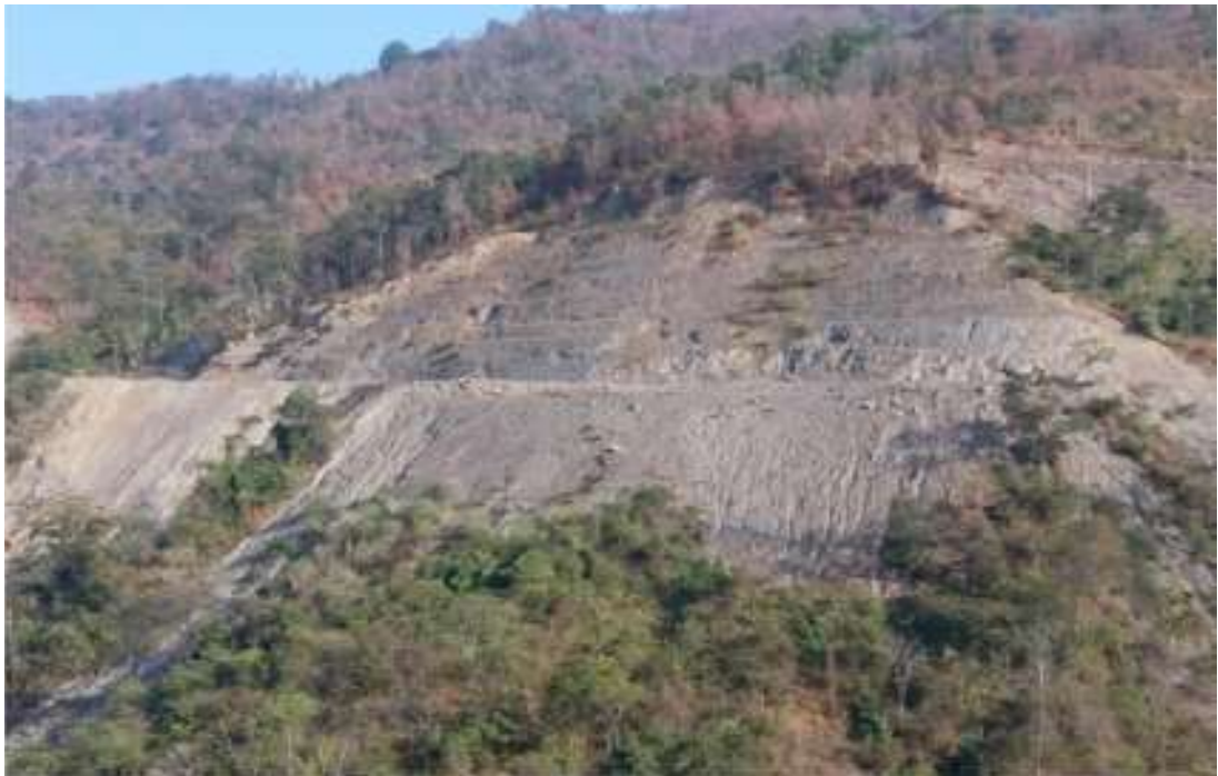
Plate 5.1.5 Landslide and rill erosion along the approach road of Kidima village due to road construction and step cutting on the top of the flow to minimize erosion
