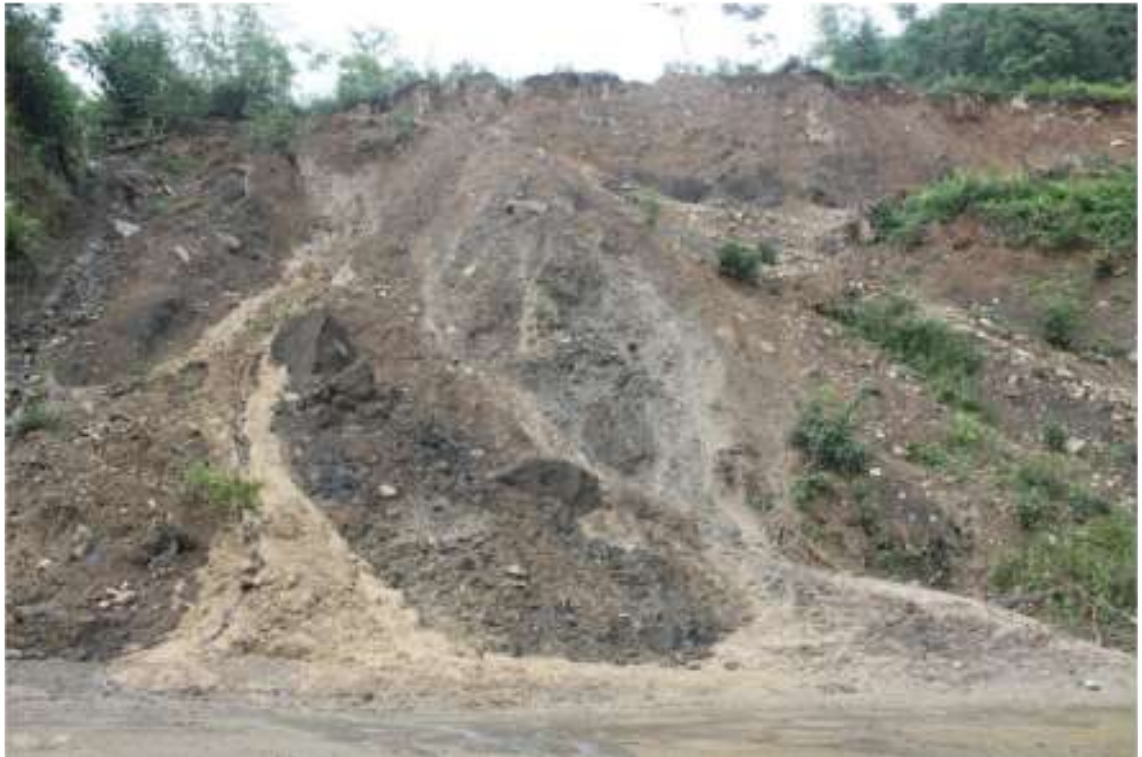
Plate 5.3.2 Landslide between Chiechama and Bosta due to improper drainage at NH 61
