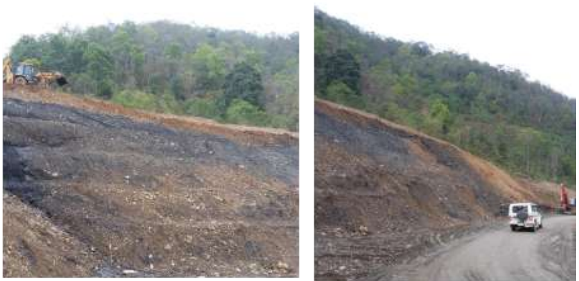
Plate 5.3.3 Cutting the top of the slide to stabilize landslide at NH 61
