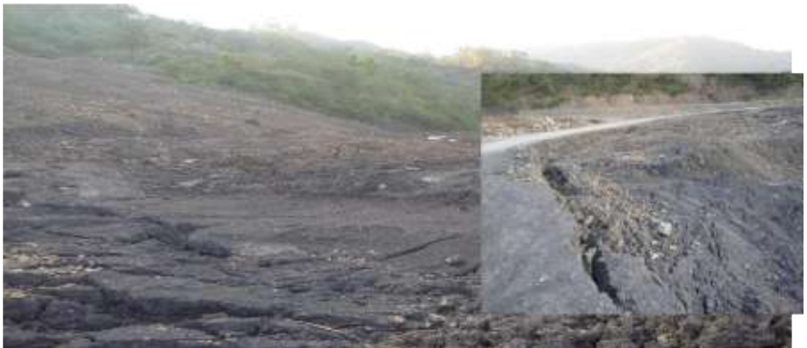
Plate 5.1.4 Landslide below Viswema village due to road construction at sensitive area
