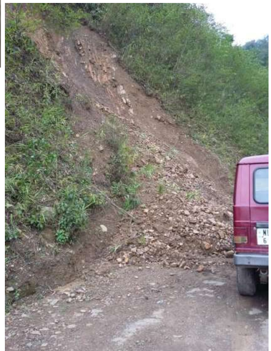
Plate 5.3.5 Rock fall along with soil along the NH 61
