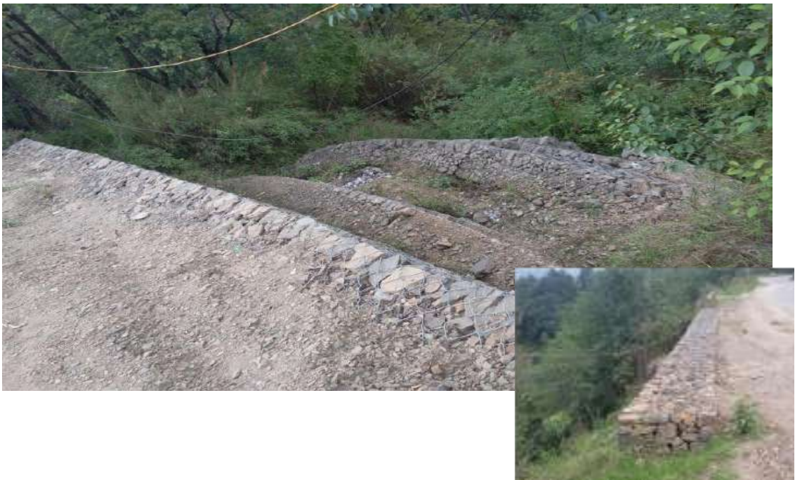
Plate 5.1.9 Retaining wall constructed at different location along the NH 39 to minimize landslide
