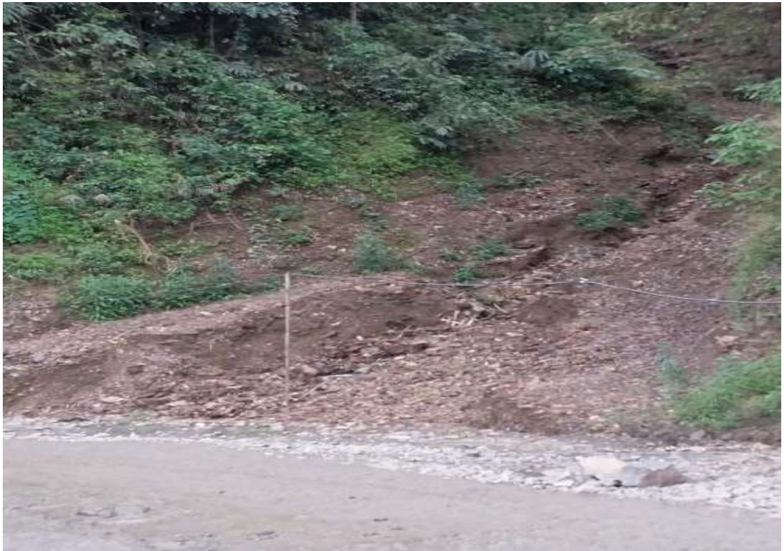
Plate 5.3.6 Drainage mud flow due loss of vegetation and settlement in the hill slope
