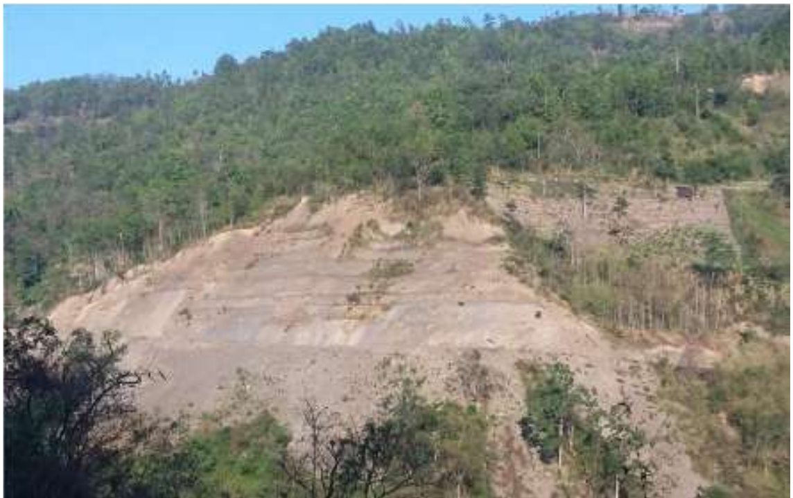
Plate 5.9 Step cutting to minimize the slope failure
