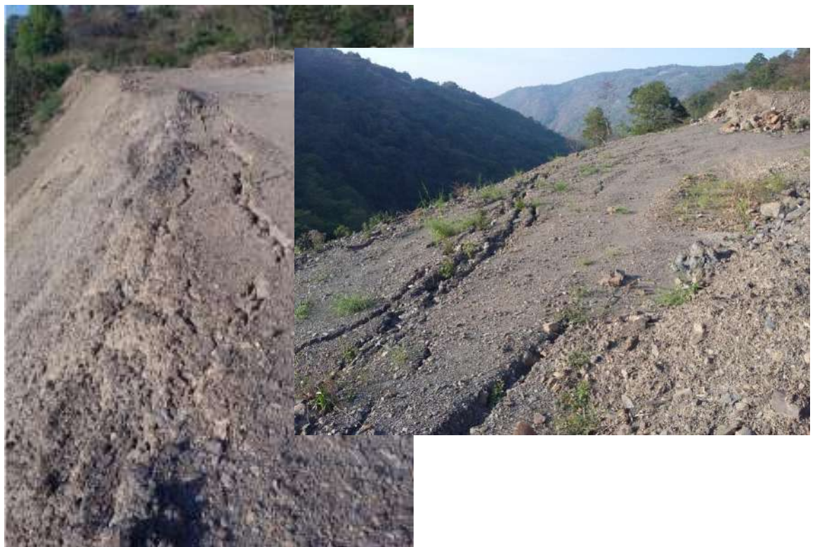
Plate 5.1.7 Cracks along a new constructed road (Viswema and Kedima approach road)
