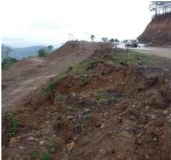
Plate 5.3.4 Mud fall and cracks at Bosta due to unscientific construction of diversion road
