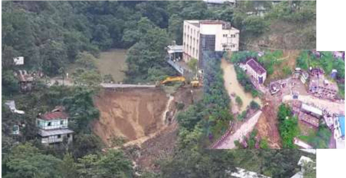
Plate 5.2.1 Arial view at Sanuorü stream erosion due to blocked of drainage along the Secretariat road
