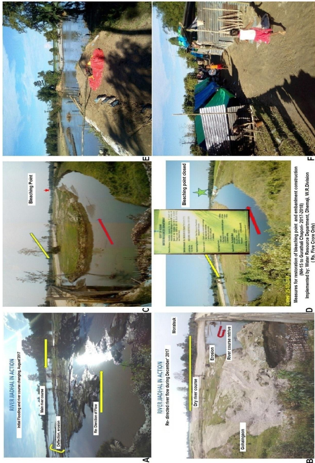
Plate. 6.4: No.3 RCC Bridge, (a) Stream flow deflected by sedimentation and flow redirected backward; (b) abounded river due to bleaching; (c) Redirected flow bleaches the embankment; (d) Bleaching point and embankment restored; (e) the bleaching point is 30 meters, and (f) Embankment used for temporary shelter.
