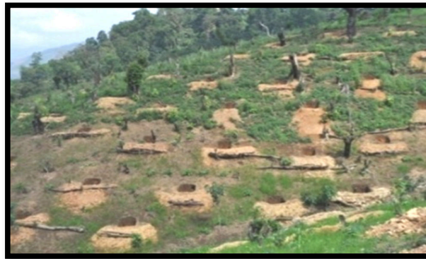
Plate 4.72: Construction of low cost water tanks
