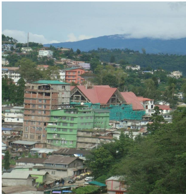
Photo plate 28. Multi-storied C3H HAZUS building type, pounding and danger of damage to nearby buildings in case of collapse.
