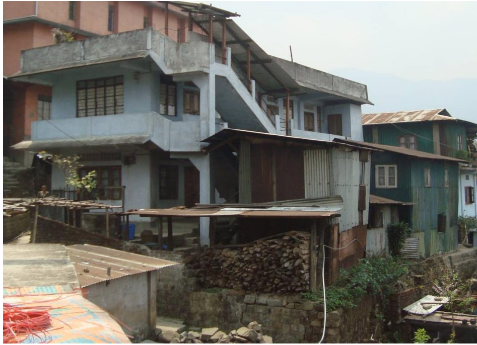
Photo plate 13. Two storey house made of RCC (class under C3L HAZUS building type)
