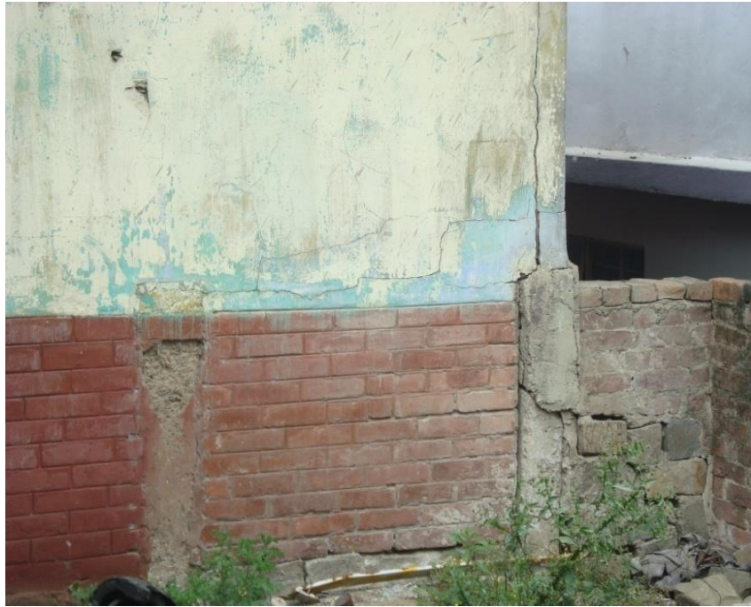
Photo plate 17. Visible cracks on the wall and columns.
