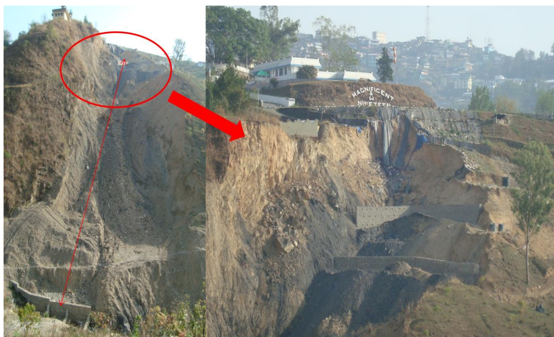
Photo plate 44. Debris flow at Ward 6, the entire length is more than 150 m.
