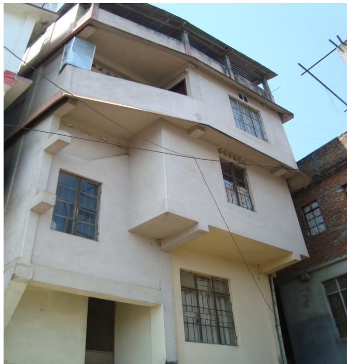
Photo plate 32. Vertical expansion of buildings causing safety issues in building design.
