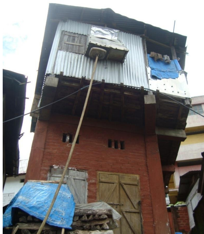
Photo plate 30. Vertical expansion of building creates unsafe structural design.
