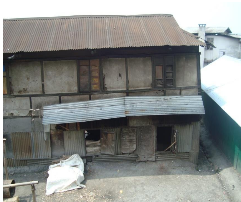
Photo plate 36. Dilapidated condition of house made of bamboo and cement building materials.
