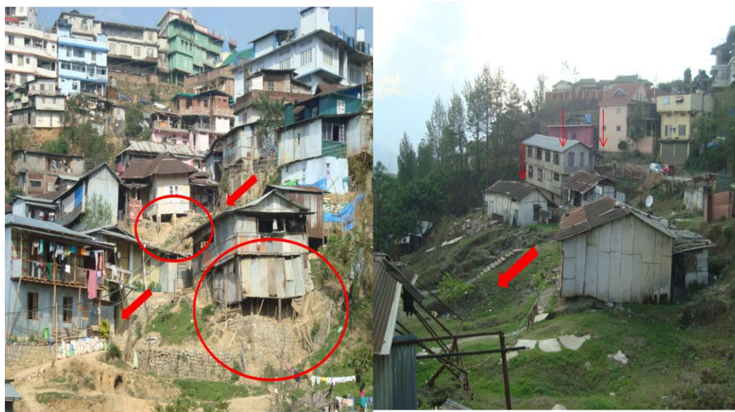
Photo plate 43. Houses affected by slide- ward 18 and ward 1. Red arrows indicate direction of slide and building weight exerted.
