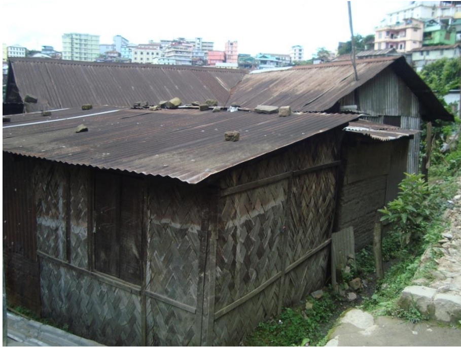
Photo plate 23. W1 HAZUS building type made of bamboo.
