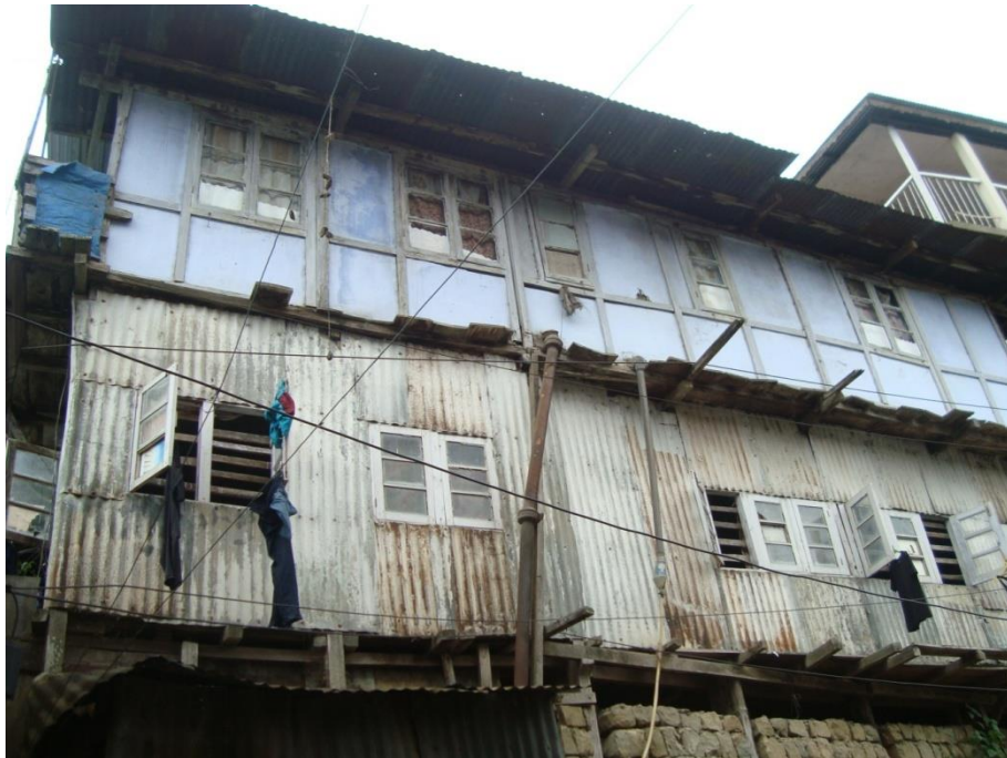
Photo plate 33. W1 building type showing a dilapidated house of asbestos, bamboo and cement construction material.
