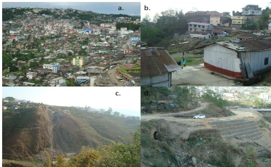
Photo plate 38. Portion of the study area- note the closely constructed concrete houses on unstable slope. b). Affected buildings in Ward no.1 of the study area. c). Landslide with an approximate length of 150 m in Ward no. 6. d). Landslide at Asian Highway (AH) 1 in Ward no. 18.
