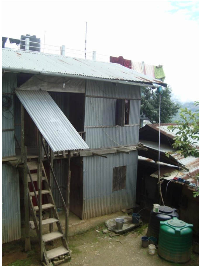
Photo plate 25. W1 HAZUS building type made of asbestos tin sheet.
