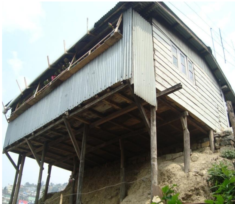
Photo plate 34. Soft storied house of W1 building type.
