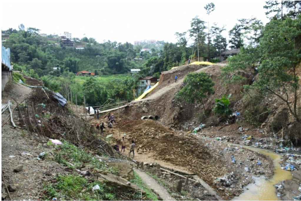
Photo plate 45. Landslide caused by breakage of culvert (New Sect. road)
