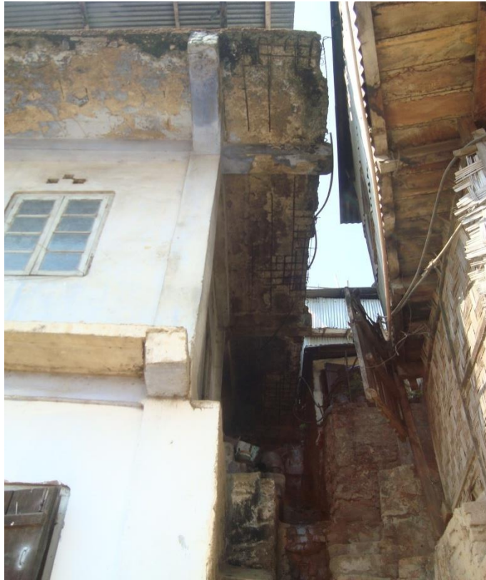
Photo plate 31. Peeling of concrete floor exposing the iron rods of the floor.
