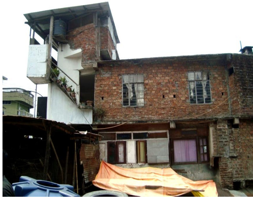
Photo plate 35. Unsafe RCC house- irregular plan.
