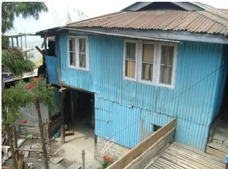
Photo plate 12. Asbestos sheet House (class under W1 HAZUS building type).
