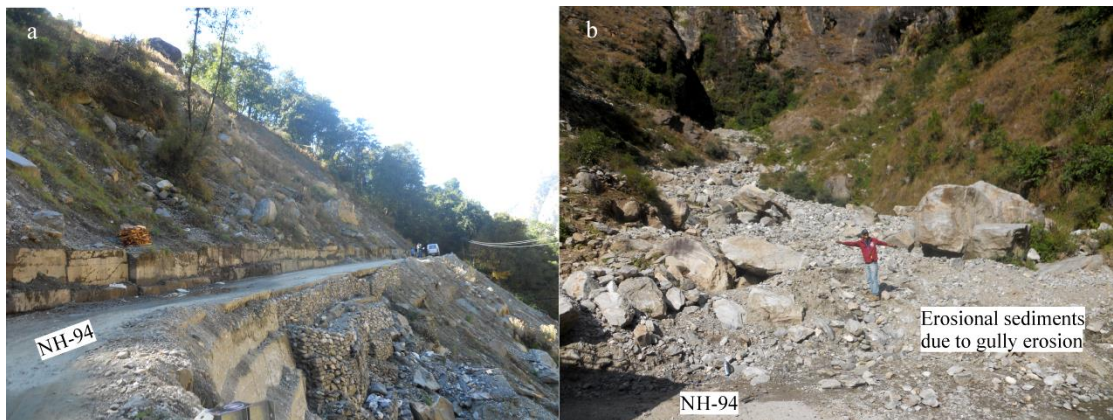
Fig. 3.6: (a) Damaged retaining wall below Wariya village; (b) Erosional deposits on the NH-94. Photograph of November 2014, prior to the disaster (November, 2017)
