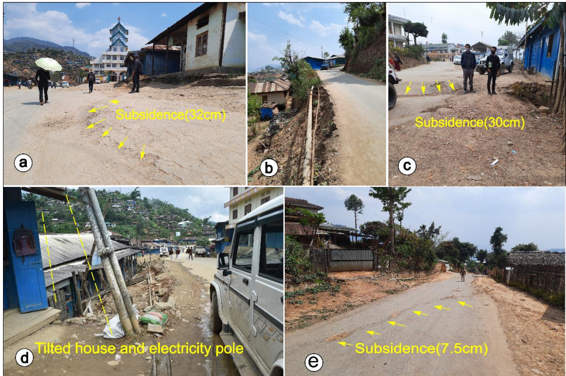
Fig 1.3. (a,b,c,d,e) Ground subsidence in different parts of the town
