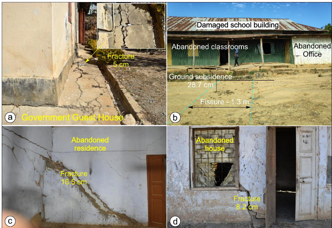
Fig 1.4. (a) Tension cracks developed inside of Government Guest House due to subsidence (b) Classrooms and office of the St. Paul School and part of the school compound affected by ground subsidence (c) Tension cracks developed inside of a residential building due to subsidence (d) House damaged due to subsidence
