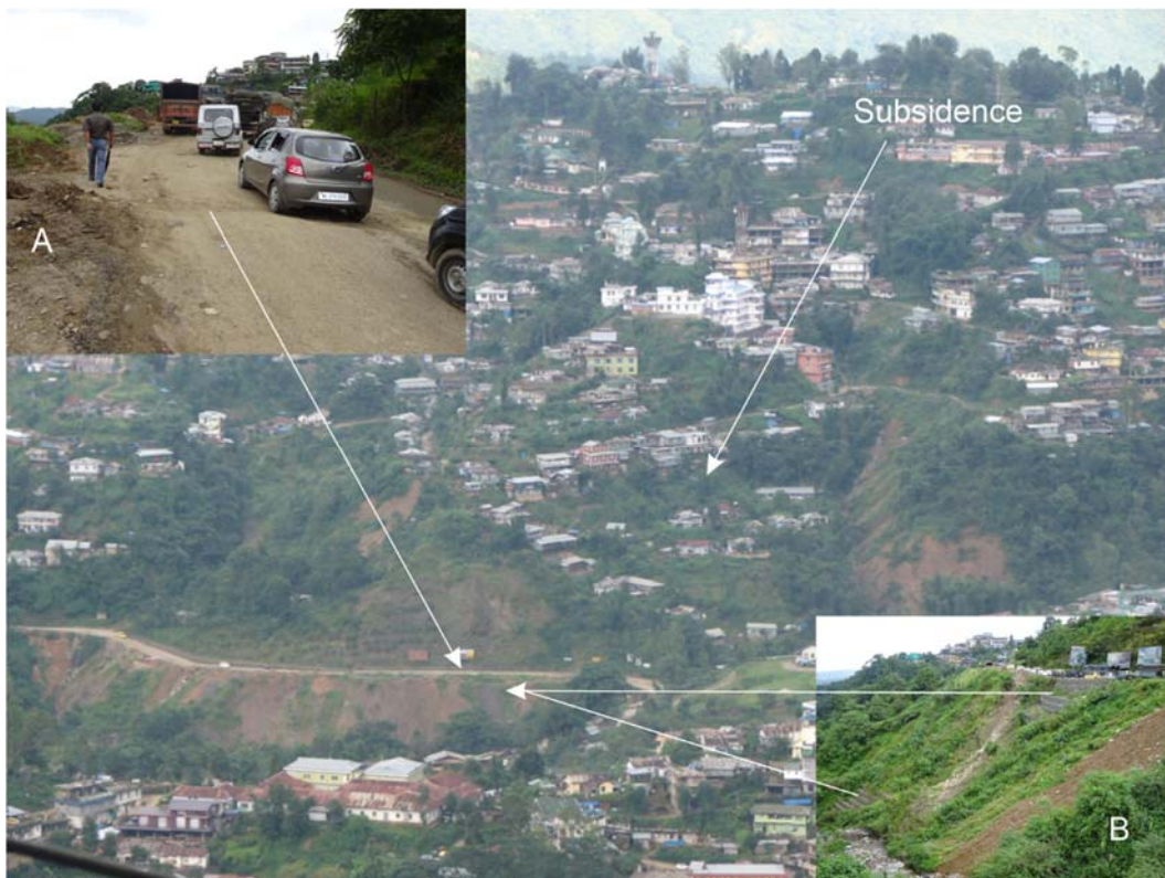
Fig. 4.1.16: Field photograph showing subsidence on the eastern bank of the stream (Inset: A - Subsidence of highway; B - Retaining walls for road support)
