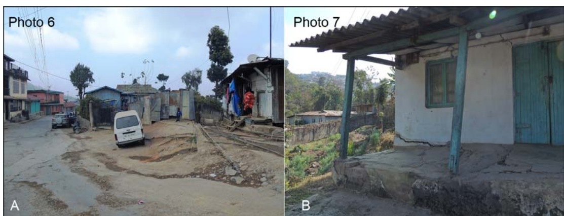
Fig. 4.2.13: A - Subsidence along the road section; B - Damaged house
