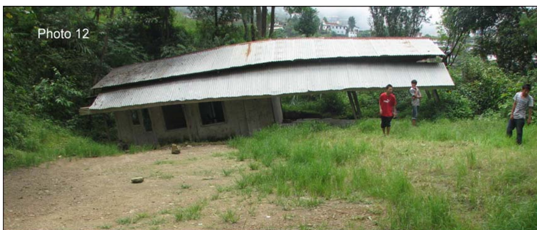
Fig. 4.1.18: House damaged due to differential settlement (Slip zone 1)
