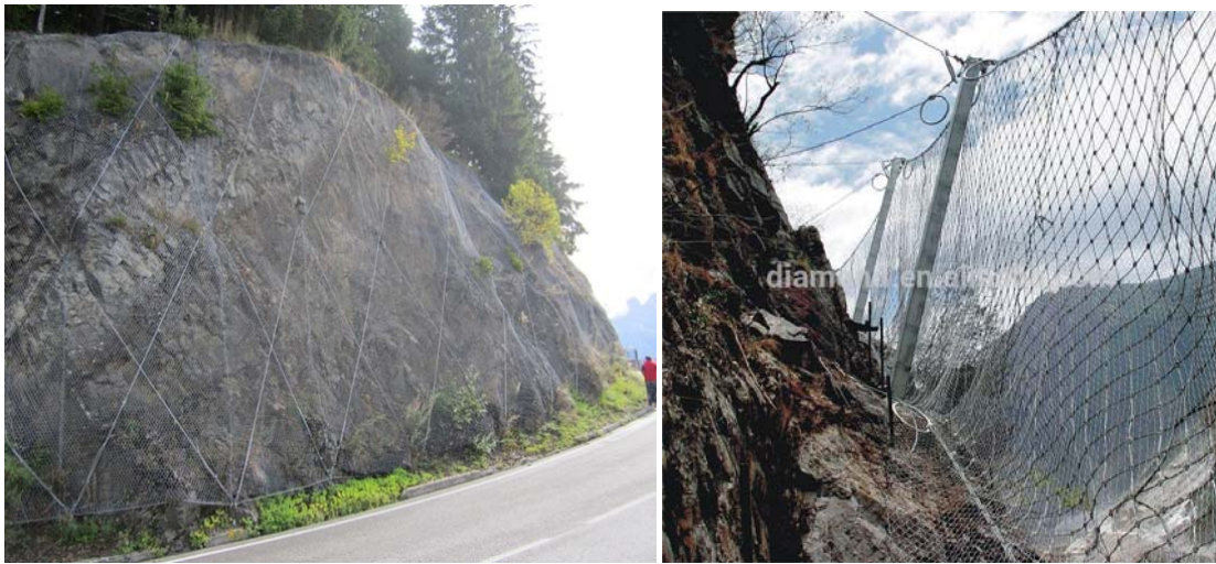
Fig. 5.1.5: Wire-mesh slope protection / Cable-net slope protection (Representational)
