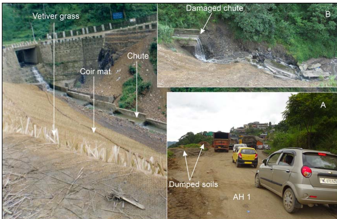
Fig. 5.1.2: Mitigation measures taken up during 2005-06 (Inset: A - Soils dumped along the highway; B - Chute damaged)
