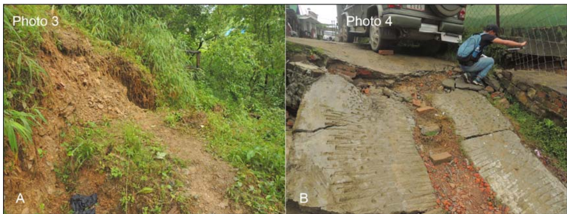
Fig. 4.2.11: A - Tension crack developed on the slope; B - Road damaged due to subsidence
