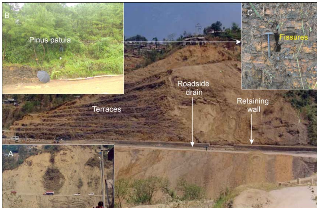
Fig. 5.1.1: Previous mitigation measures in the weak zone (Inset: A - Landslide during 2005; B - Needle pine plantation; C - Open fissures)
