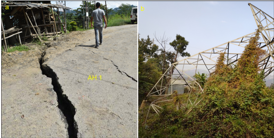
Fig. 4.3.3: Effects of the landslides - a Large fissure on the highway at the eastern edge of the slide zone; b Collapsed pylon (major support for power cables to Kohima)
