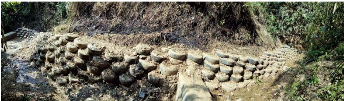
Fig. 5.1.4: Used tyres forming a protective wall against toe erosion (Representational; Source: Mr. Sukho Movi)
