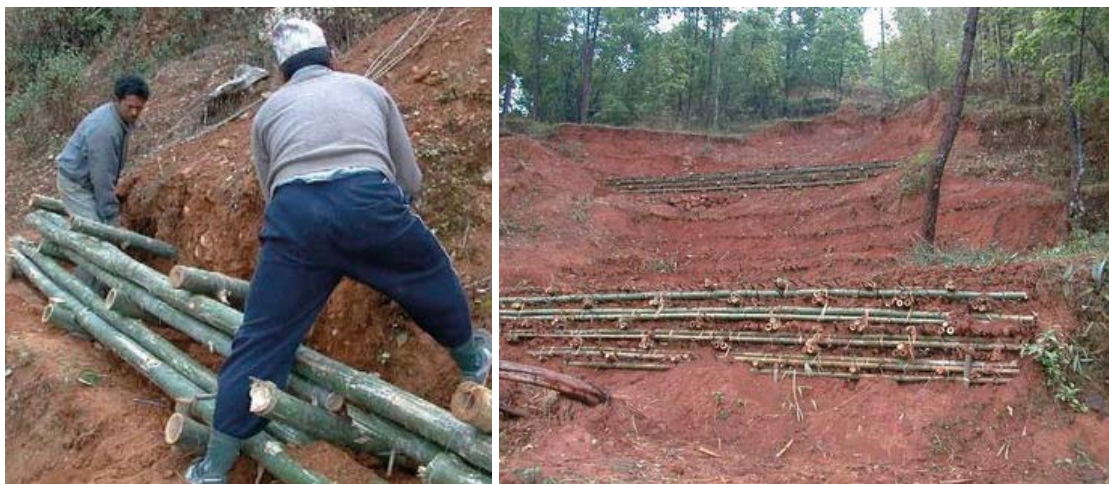
Fig. 5.3.4: Crib wall retaining structure made of bamboo (Source: Rauch et al., 2002)
