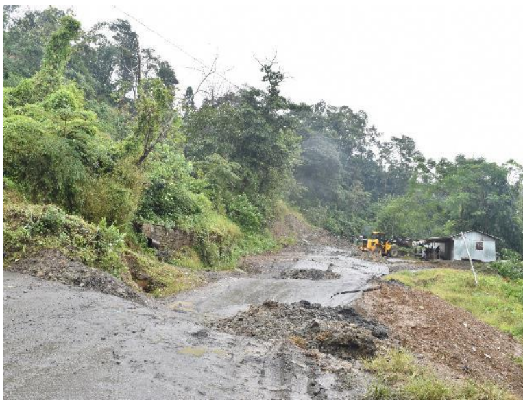
Fig. 6.1.2: Swelling of road sections along NH 2 at Meriema due to clayey soils
