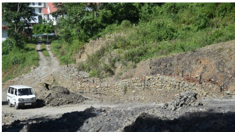
Fig. 6.2.3: Gabion wall at Meriema slide zone
