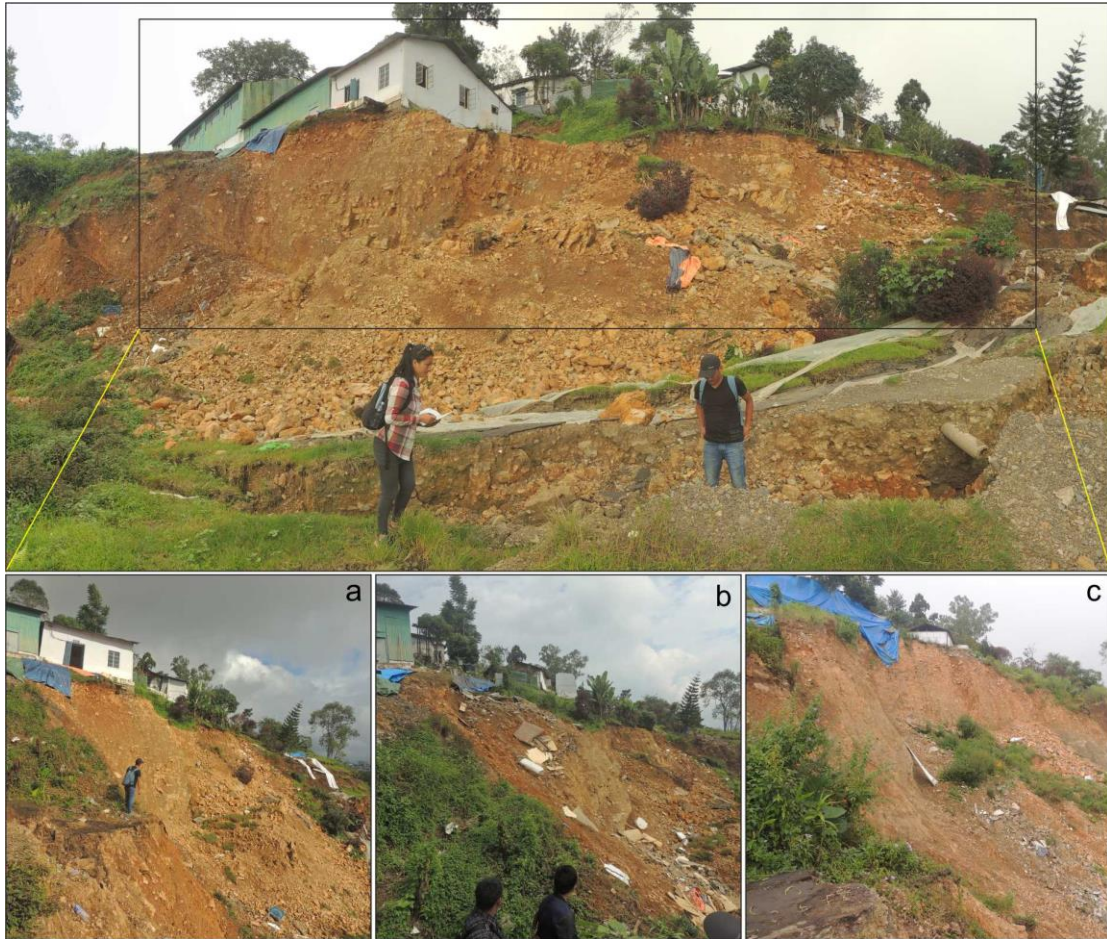
Fig. 6.1.4: Fractured shale at crown (Box - unstable scarp) in Peraciezie, 2018. Changes at crown: a) 30 th August 2018; b) 13 th September 2018; c) 31 st August 2019
