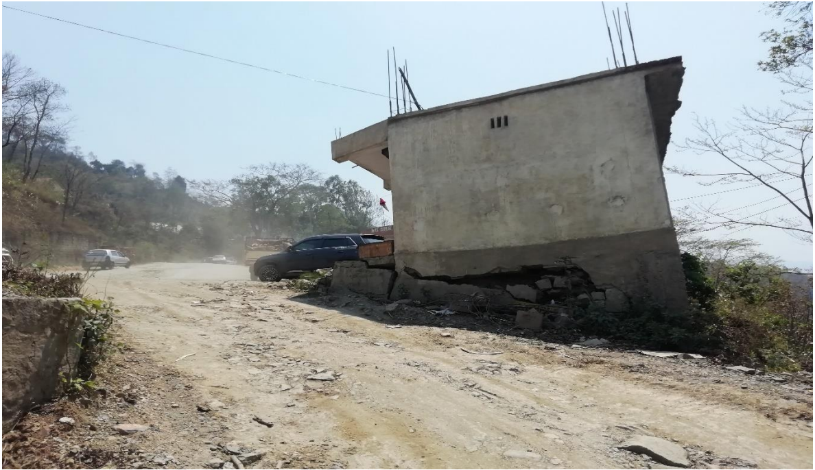
Plate 12: A subsidence zone along the Mereima village resulting in cracks and fissures in the nearby constructed buildings and roads
