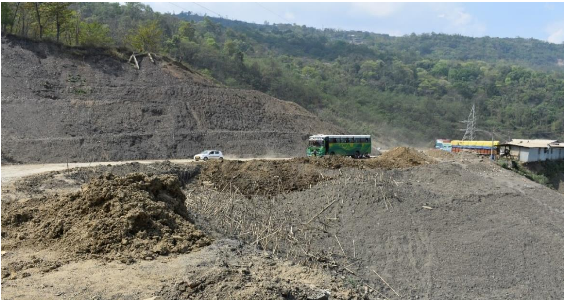
Plate 4.6: Dumping of road cut materials along the NH-29 highway due to road construction which is responsible for downstream deforestation, killing of vegetations and drying up of springs.
