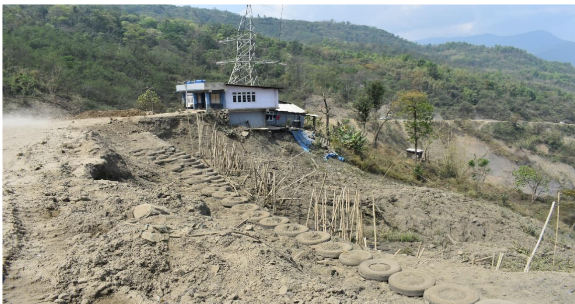
Plate 4.7: Indigenous treatment of landslide by bamboo hammering and other measures for checking of land degradation and soil erosion downslope of NH-29.
