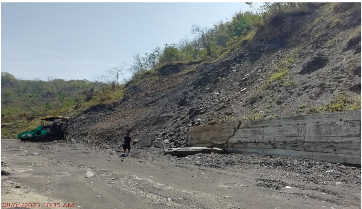
Plate 13: Massive road cutting along the NH-29 (Zubza) causing numerous landslides and rockfalls
