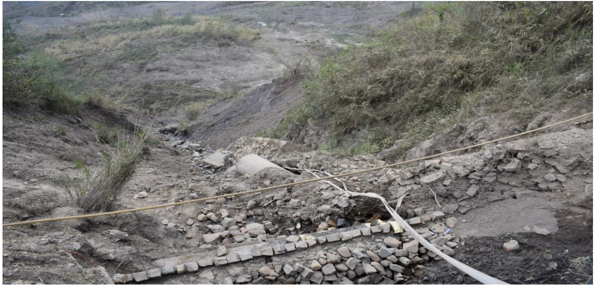
Plate 4.2: The collapsed retaining wall in section 2 of NH-29 selected 2km stretch, Kohima
