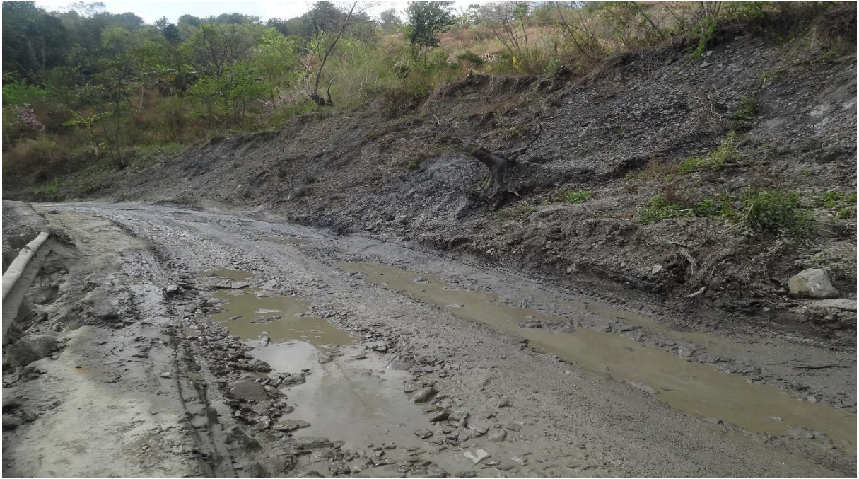
Plate 14: The southern stretch of NH 29 (Phesama) upslope evident of land failure
