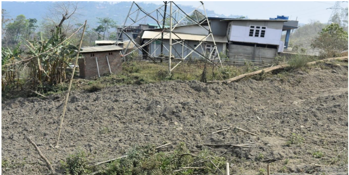
Plate 4.1: Tilted electric posts and houses and dumping of landslide materials in the selected section 1 of NH-29 selected 2km stretch Kohima
