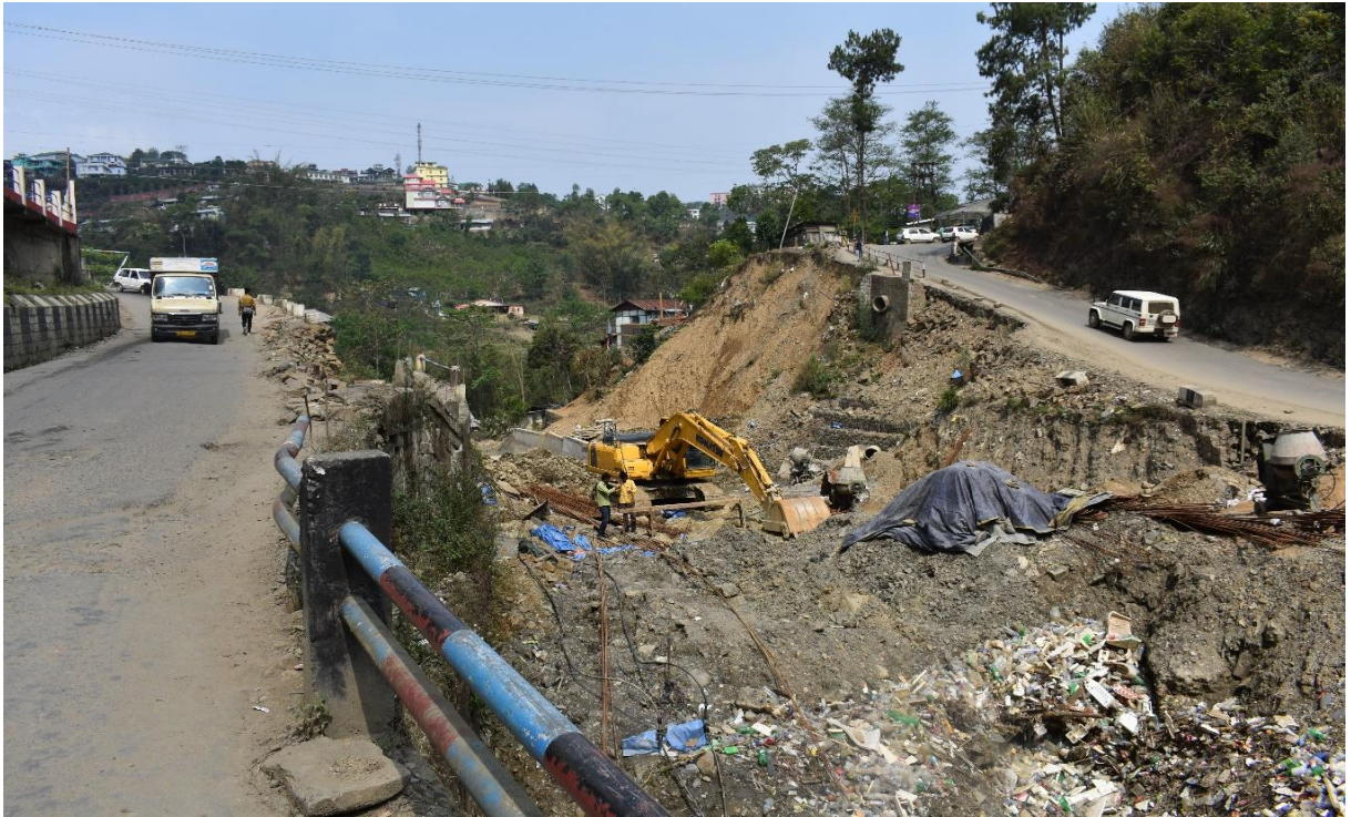
Plate 6: The infamous Sano ru landslide due to the presence of a fault accompanied by heavy monsoonal rains. This watershed is categorised under the highly stressed ecology
