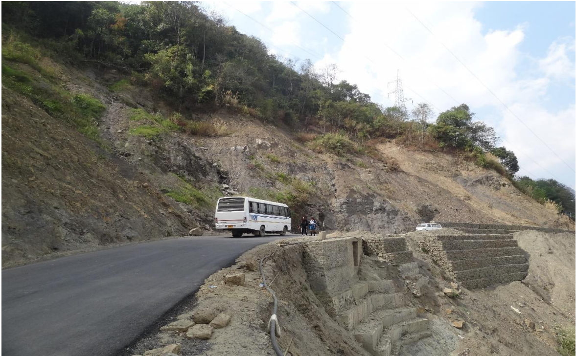
Plate 16: Retaining walls built along the highway passing through Phesama village to combat the subsidence and land creeping
