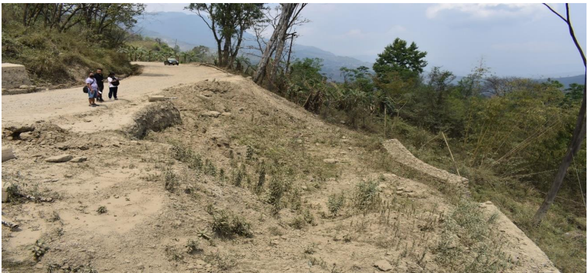
Plate 4.5: The downslope and upslope of section 4 of NH-29, Kohima sliding down with tilted bamboo and trees.
