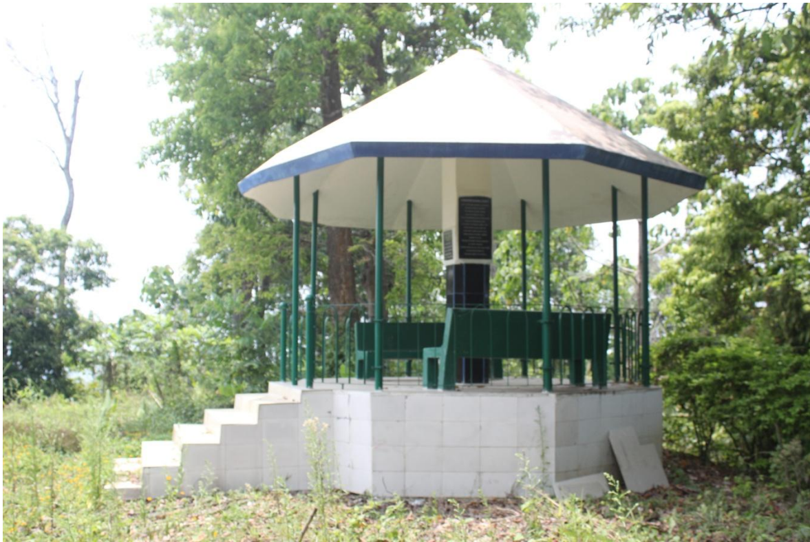
Plate 17: A view of the Rest House located atop Maipang Site's hill
