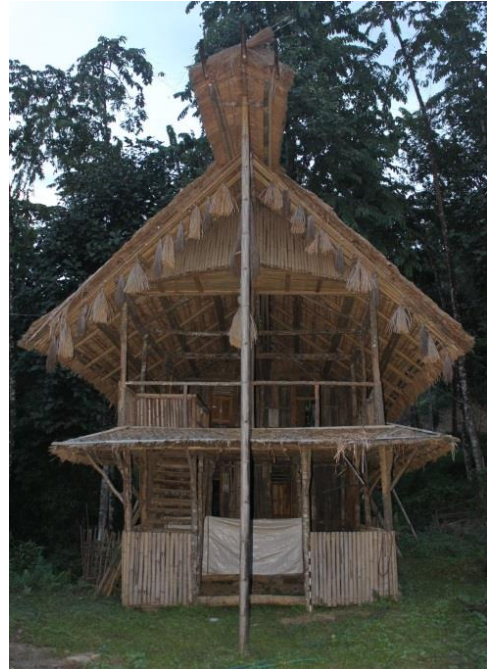
Plate 62 & 63: Raised platform and stilts as the foundation, which helps protect the home from dampness and pests. (Ungma village and Changtongya Old).
