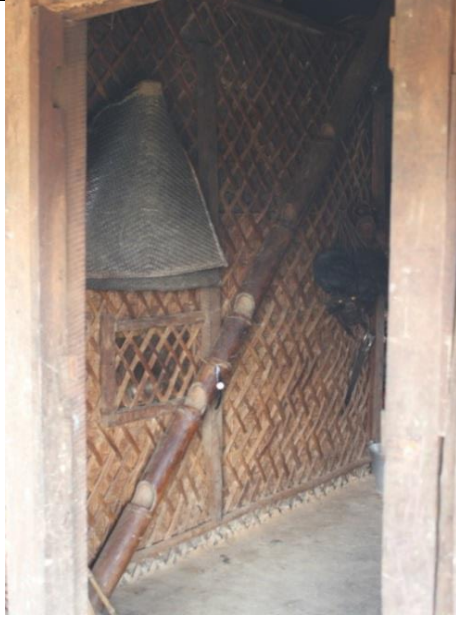
Plate 14: Bamboo ladder ( Kavu Lashe ) – an essential architectural element in traditional domestic construction, enabling vertical mobility during construction and daily household activities.
