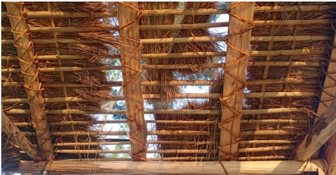
Plate 79: Imperata cylindrica (thatching grass) and bamboo are traditionally utilized to create roofs that are resilient against the heavy monsoon rains.
