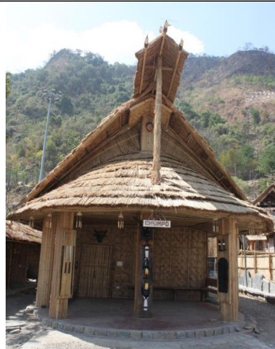
Plate 37: Traditional Lotha tribe Chumpo , a circular structure with a conical thatched roof, bamboo walls, and buffalo skulls on the roof ridge.
