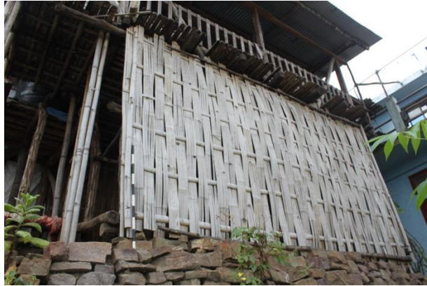
Plate 82: Stones provide a solid base for the wooden or bamboo stilts that support the homes.
