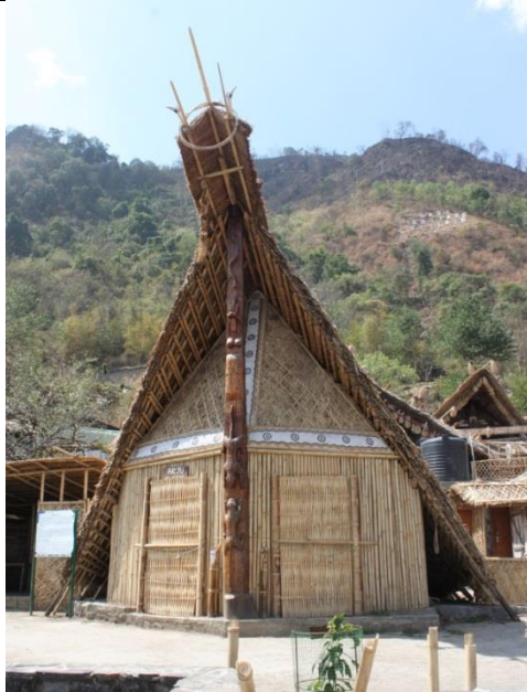
Plate 33: Traditional Ao Naga Arju ( morung ) featuring a steep thatched roof, intricate bamboo weaving, and symbolic carvings (a bamboo spike crowns the apex, symbolizing strength and identity, while the main pillar, adorned with animal motifs, reflects the owner's achievements).
