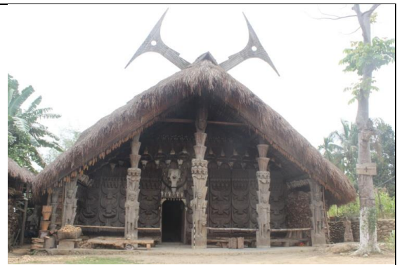
Plate 102: Chakhesang Naga architecture, linked to the Feast of Merit, features gable horns (Donors who complete rituals earn the right to wear the lichira/thüpiikhü shawl, erect monoliths, and build homes with elevated gable horns)
