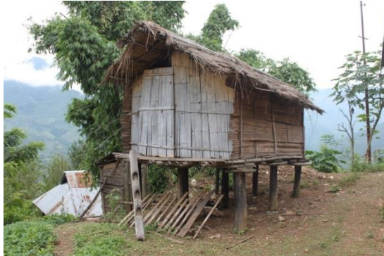
Plate 49: Separate raised hut granaries outside the house (Phelungre, Kiphire District) and a granary bamboo basket inside the house (Mesulumi, Phek District) protect harvested grains from pests and moisture.
