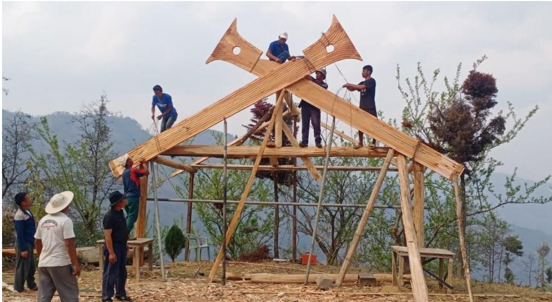
Plate 83: Community participation in traditional Naga house construction.
