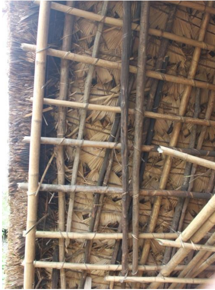
Plate 65 & 66: Common roofing used such as Trachycarpus fortunei (Arecaceae) and Imperata cylindrica (thatch grass).
