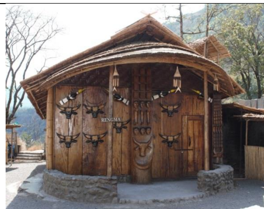
Plate 41: Traditional Rengma morung with a carved thatched roof for insulation and rainwater runoff (intricately carved wooden panels featuring mithun and buffalo motifs).
