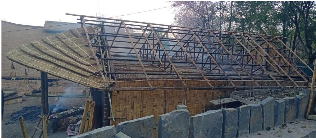
Plate 64: Bamboo is also integrated as a skeletal framework between timber and thatch.
