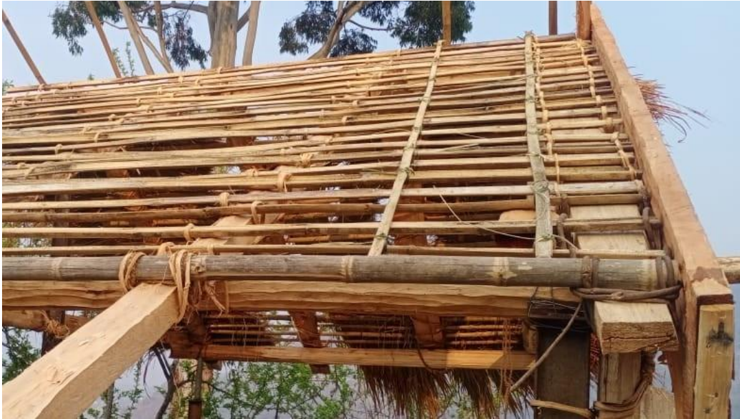
Plate 80: Lashing techniques that use natural fibers (Local name buwu ), rattan strips, or vines to bind bamboo and timber components together.
