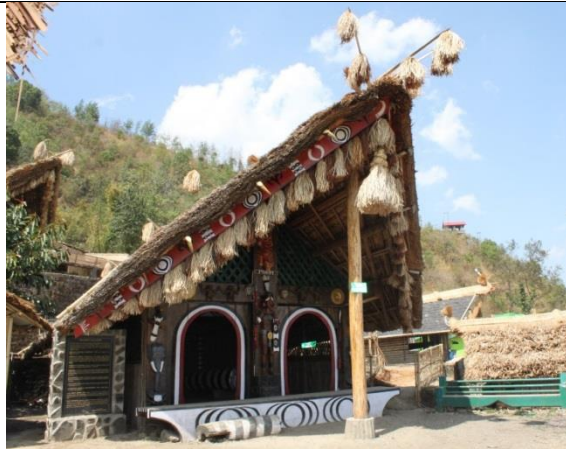
Plate 39: Traditional Phom morung , featuring a steeply sloped thatched roof adorned with decorative tassels and bold tribal patterns (carved wooden pillars and an arched entrance, elevated ridge with wooden poles and straw bundles).
