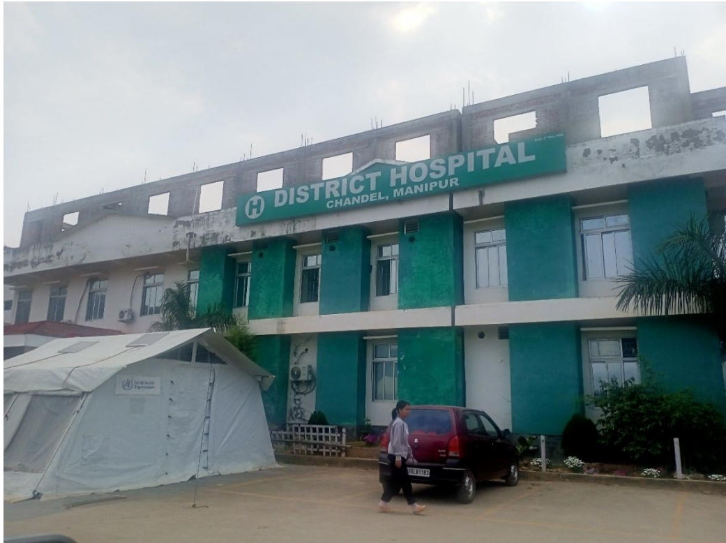
Photo Plate 30: District hospital
