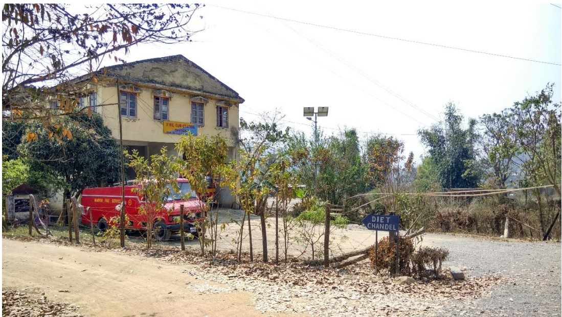
Photo Plate 31: Fire Sub-Station at Nahtham village.
