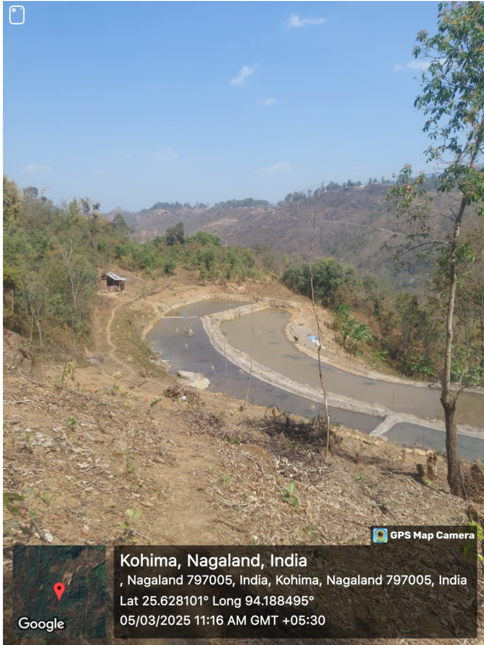
Photo Plate 4 Fishery Pond in Kohima District. Photos taken for validation of LULC.
