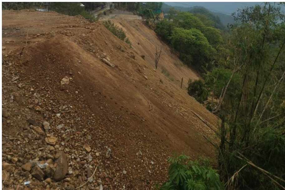
Plate 5.2: Road cut debris triggering slope instability and distorting vegetation.
