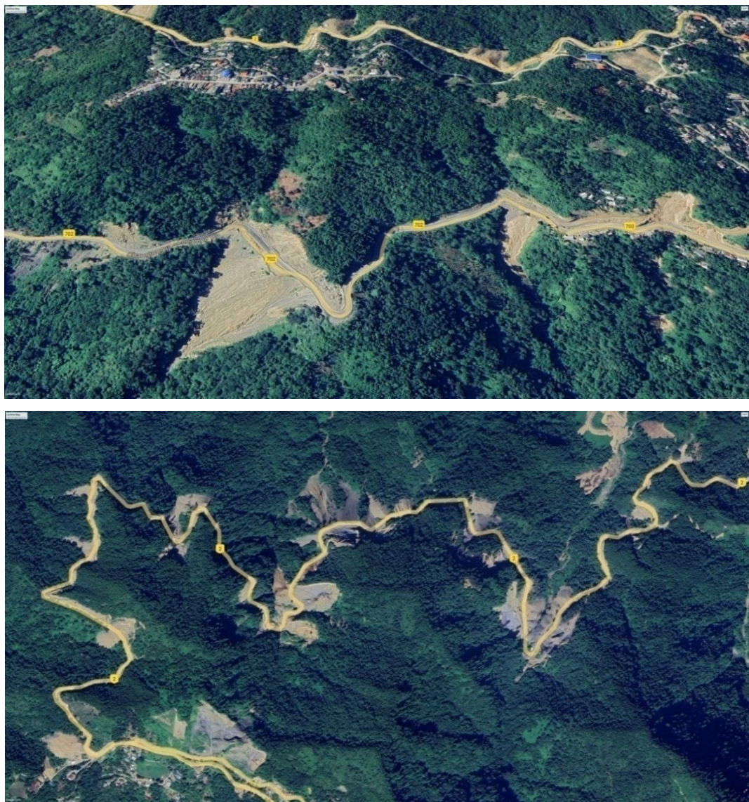
Figure 5.9: Slope failures along road-cut sections in Mokokchung District.
