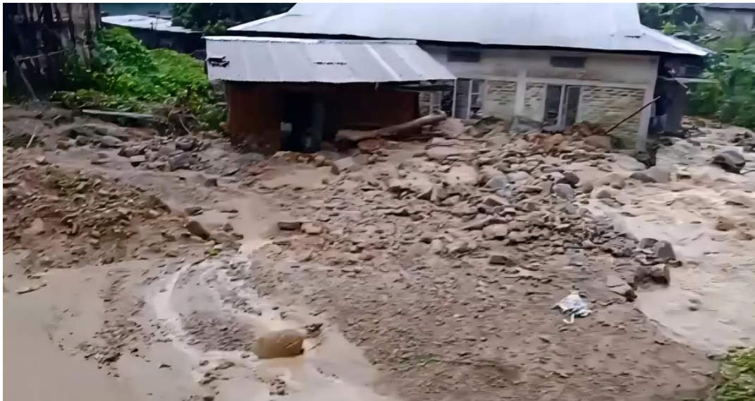
Plate 5.9: Houses exposed to debris flow during flash flood in Mangkolemba.
