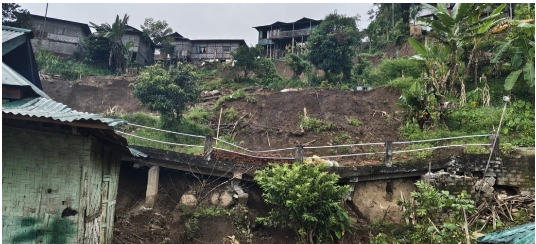
Plate 5.6: Active slope failure in a settlement, showing exposed soil and unstable terrain in Chungtia village.
