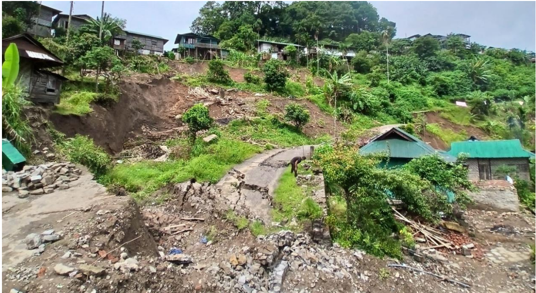
Plate 5.5: Post-landslide terrain disruption with damaged access routes and altered slope in Chungtia village.
