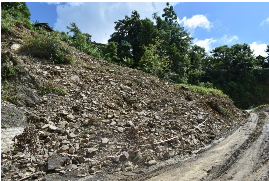
Plate 5.7: Deep seated, debris slide involving the downward movement of weathered rock and soil mass along a slope failure.
