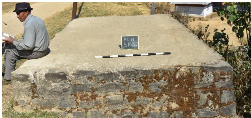
Plate 79: Recently constructed Bam /sitting platform, Poilwa village
